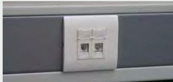
Socket for data transfer / Telephone
