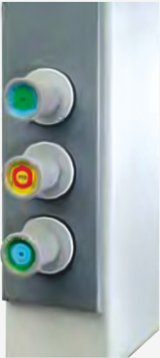
Fume hood valve
